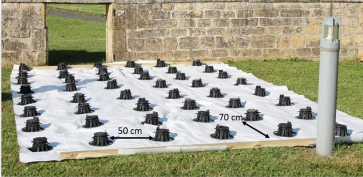
> Start by laying the geotextile tarpaulin over the entire length of the site. This cover will prevent the growth of weeds below the terrace and will save you from weeding between the blades.
