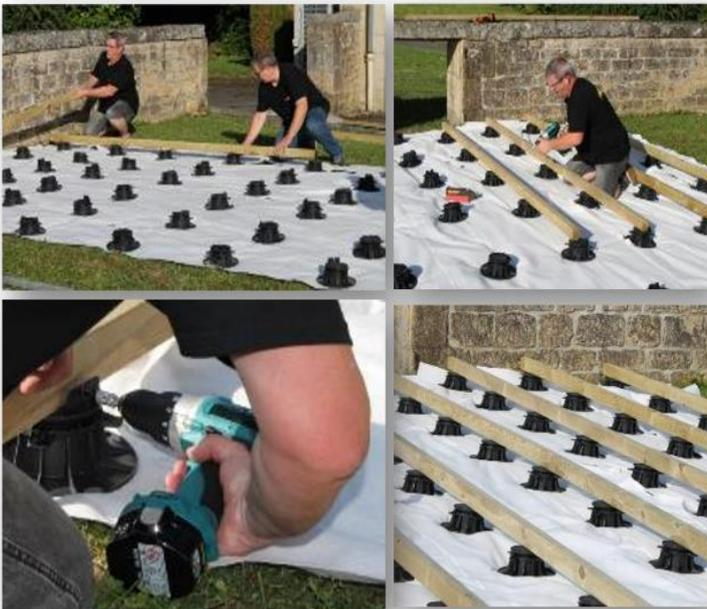
> Place the joists on the lines of pedestals and secure them with 5x40 stainless steel ROCKET screws.
